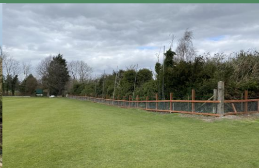
Top rails to be added and post to be levelled off.
